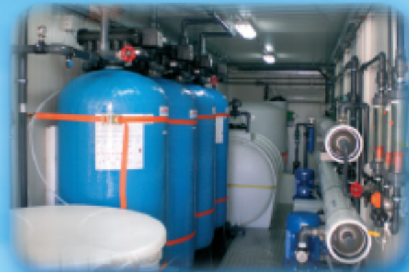
FARMACEUTICALS CAPACITY: 4 m 3 /hr FEED WATER QUALITY: BRACKISH WATER PRODUCT WATER QUALITY: ULTRAPURE
