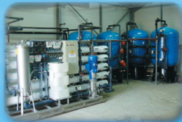
FOOD INDUSTRY (ROUMANIA) CAPACITY: 720 m 3 /day FEED WATER QUALITY: 1000 ppm TDS PRODUCT WATER QUALITY: 250 µS/cm
