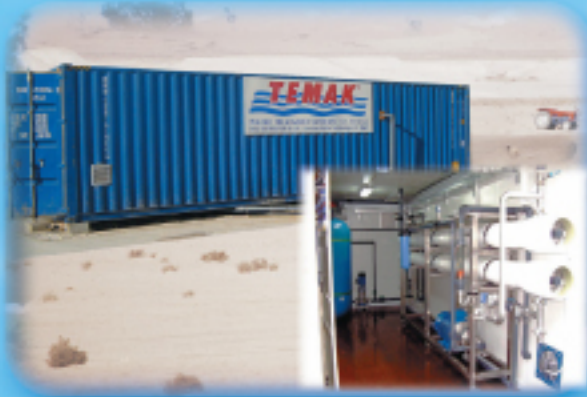
WATER FOR CEMENT PRODUCTION (UNITED ARAB EMIRATES) CAPACITY: 200 m 3 /day FEED WATER QUALITY: SEA WATER PRODUCT WATER QUALITY: 500 ppm TDS
